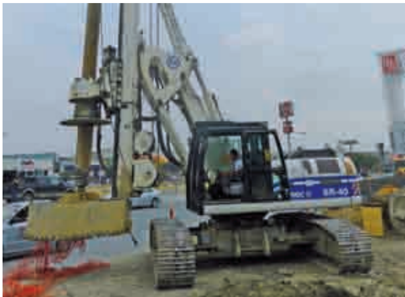
The SR-40 equipped with 2,400 mm diameter bucket.
