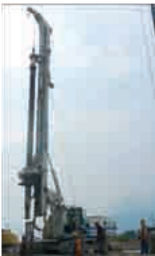
The Soilmec SR-30 equipped with cylinder crowd system.
