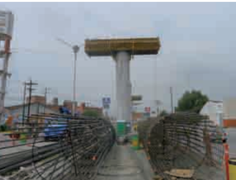
The Line 3 pier structure and the drilled shaft reinforcing cage.
