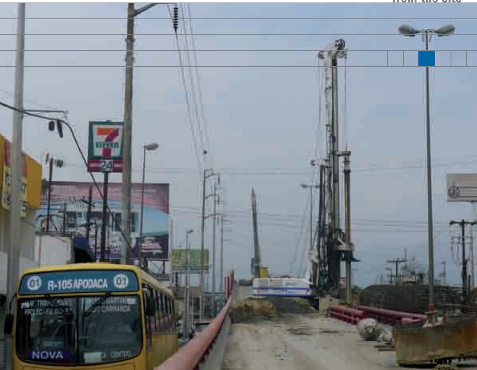
The Soilmec SR-70 working on a road overpass.
