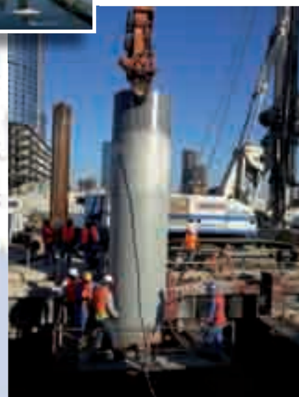
Soilmec SR-80 is working to build foundation piles for four new bridges in Abu Dhabi , UAE
