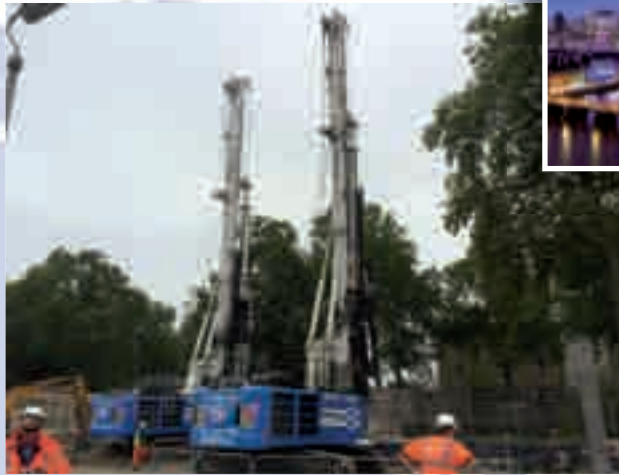
Two new generation Soilmec rigs, an SR-90 and an SR-75 , at work in Chelsea, London , UK
