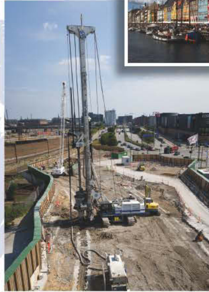
Soilmec SR-100 in action for Cityringen Metro Project, Copenhagen
