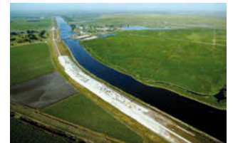
Herbert Hoover Dike near lake Okeechobee, Florida (USA).
