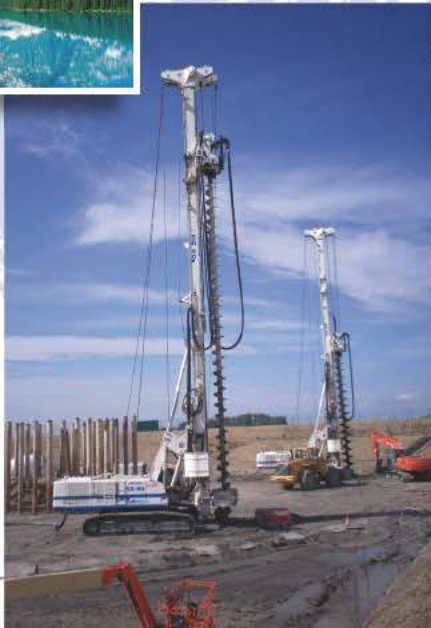
Soilmec SR-90 in CFA configuration at work in Canada
