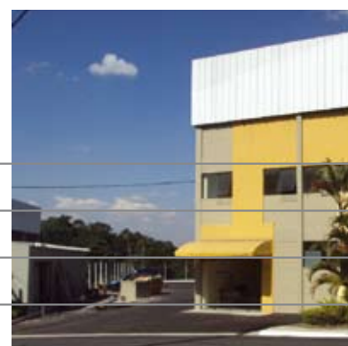
External view of the production unit.
