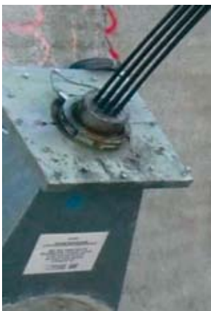
The VSL anchor system was fitted complete with load monitoring collars.
