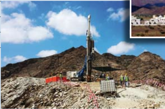
Soil investigation with Soilmec drilling rig for the "Sifah Road Project", Oman
