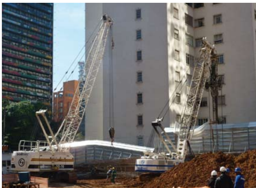
The SC-70 crane with BH-8 hydraulic grab at work in Barra da Tijuca building infrastructures for the forthcoming Olympics.
