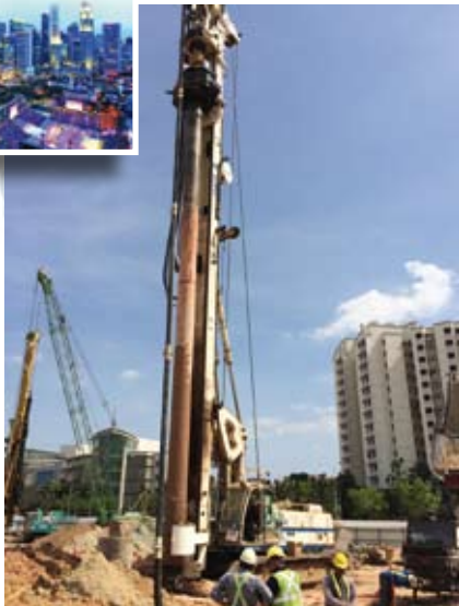
The first Soilmec machine in CSP configuration went into action, Singapore
