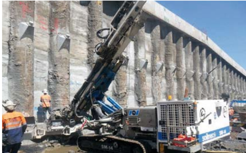
VSL's own Soilmec SM-14 drilling rigs carried out most of the drilling work.
