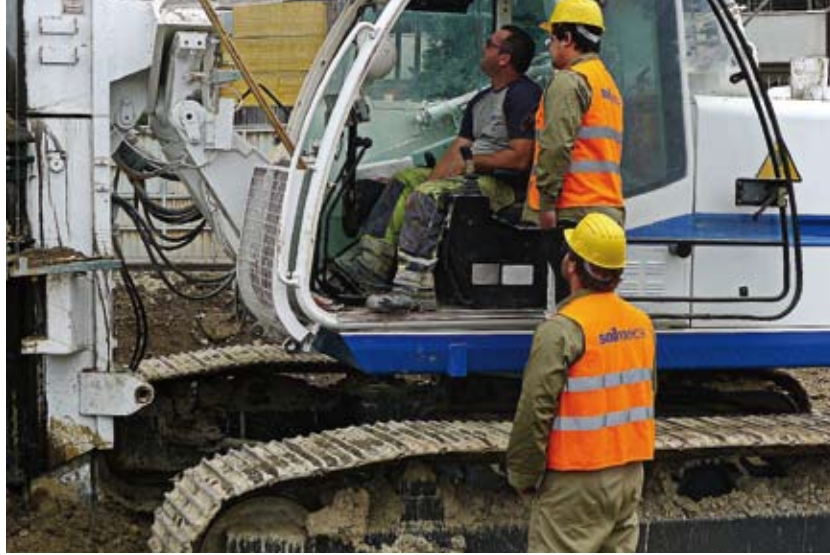
Operators can follow the different pile execution phases thanks to DMS monitoring system.
