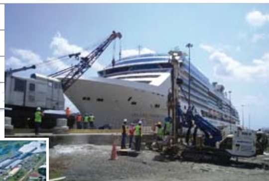
Soilmec SM-8 in action for subsequent injections performed for the Panama Canal expansion Project
