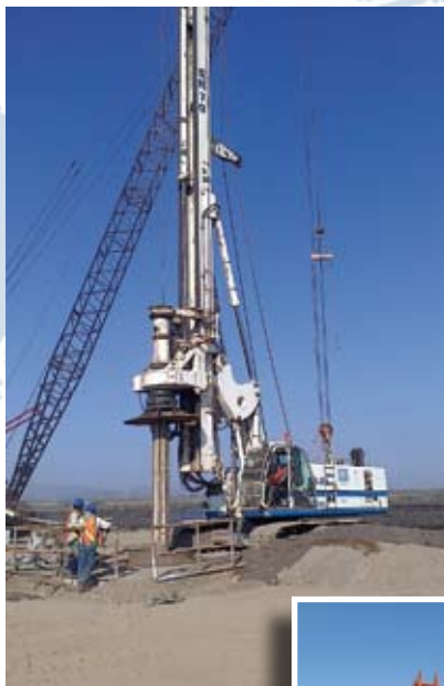
Soilmec SR-70 drilling rig at work near Lázaro Cárdenas, Michoacán, Mexico
