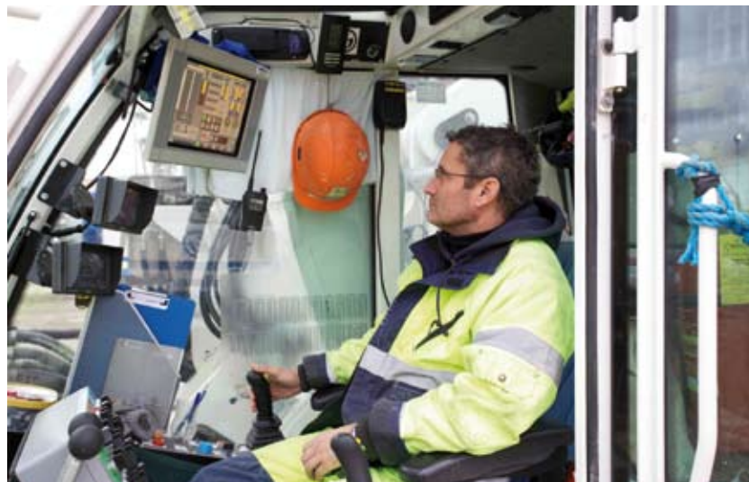
A Trevi worker uses Soilmec’s Drilling Mate System to monitor the hydromill diaphragm wall construction in Copenhagen.
