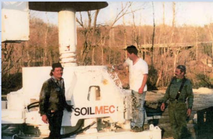
Workers christen Hub Foundation's new R-622 in May, 1992.
