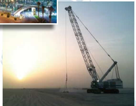
Dynamic compaction with Soilmec SC-120 in Damman, Saudi Arabia
