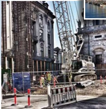
Cage positioning with Soilmec SC-100 in Copenhagen , Denmark
