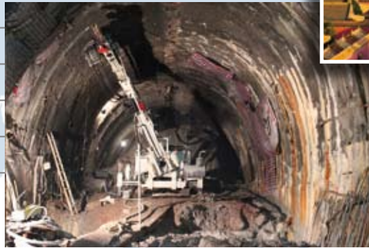
Soilmec ST-20 positioner for tunnel consolidation in action in China
