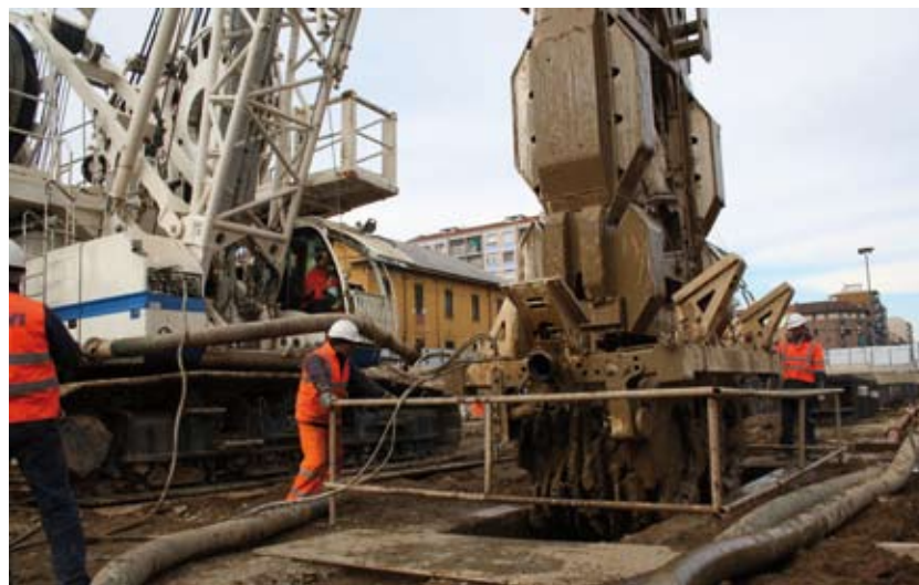
Hydromill positioning into the trench.
